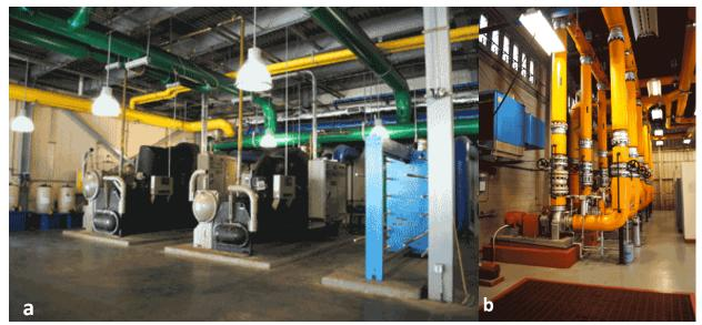
Figure 4: (a) The chillers inside the South Heating and Cooling Plant [8], (b) Part of the boiler system inside the South Heating and Cooling Plant [8]
